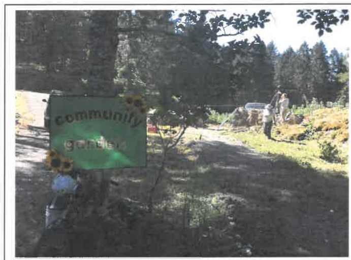
Highlands Community Garden – Fence Construction, August 2017
